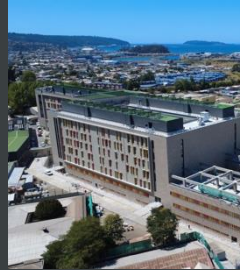
Hospital Hígueras de Talcahuano 61.659 m 2
